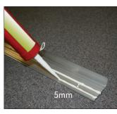
Apply 5mm bead to the underside of the profile, 2 lines for Single and 3 for double channel.
