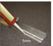
2 Apply 5mm bead to the underside of the profile, 2 lines for Single and 3 for double channel.
